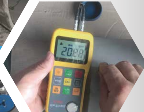
UT for Wall Thickness
